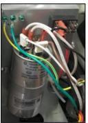
Step 4 – Crimp the appropriate spade terminals onto the STA01 system as needed and as instructed in the STA01 installation manual. Feed the STA01 cord between the capacitor bracket & fan motor bracket. Connect the Air STA01 (ASY-364-X36-UL) wires as follows:
